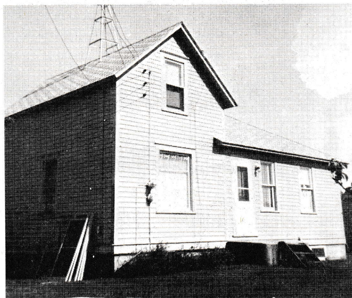
Thomas and Anna Wilebski Home Once located on the farm in Wanger Township, it was later moved to the city of Argyle, Minnesota
