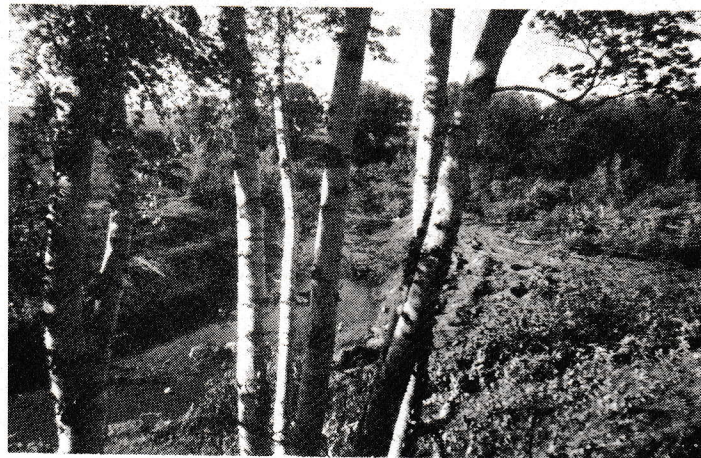
Tamarac River bed as work began -- 1973
